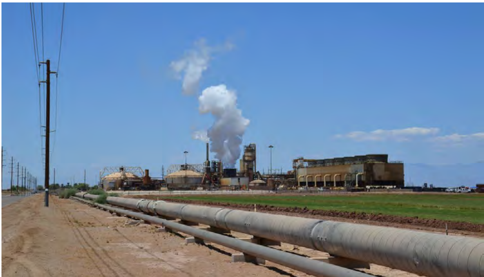
Fig. 1: Geothermal power plant, Imperial Valley, California/United States (Sven Stremke)
